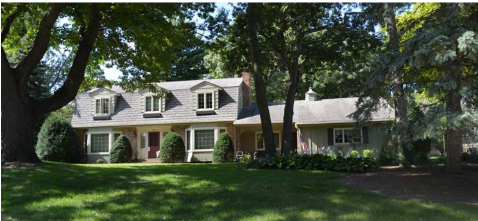
The Gambrel Roof Colonial Revival was a popular revival style as seen here at 1731 Reservoir Boulevard.
