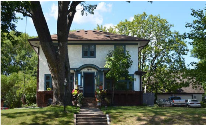
This house at 3840 Reservoir Boulevard displays Prairie influences in its stucco exterior and low-pitched roof with wide overhanging eaves. This property also has an American Foursquare appearance.
