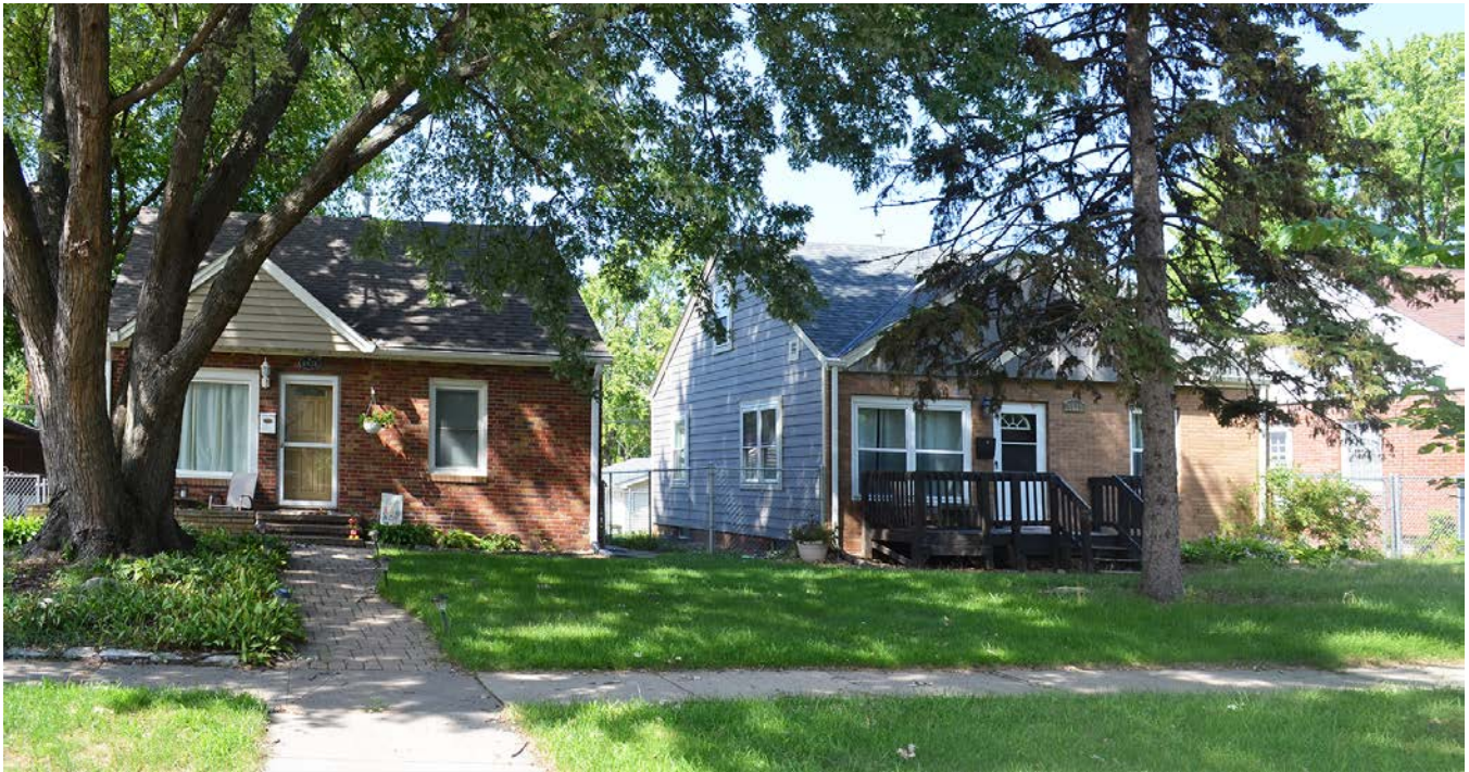
Brick-faced cottages in the 4900 block in northern Columbia Heights.
