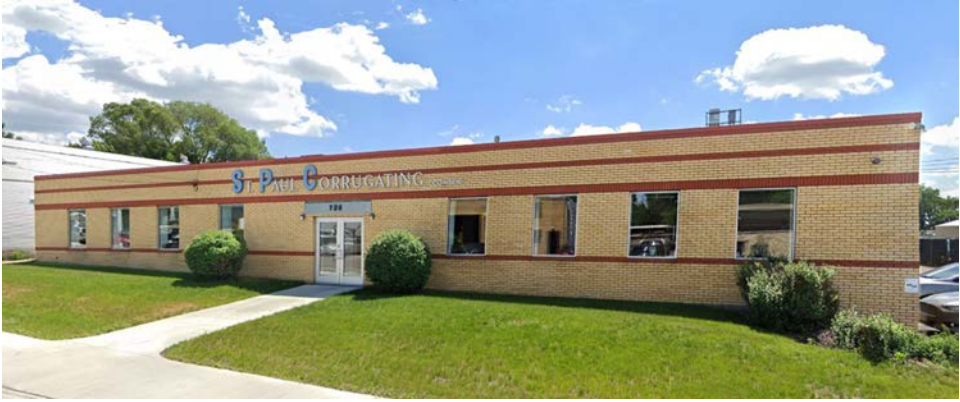
The St. Paul Corrugating Company at 700 39th Avenue NE specializes in the fabrication of corrugated metal products.
