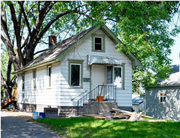
This cottage at 4340 2nd Street NE displays all the identifying features
