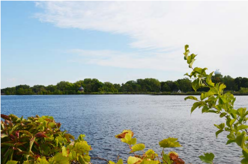
The open reservoir looking to the northeast. One of the gatehouses can be seen in the distance in the center left.
