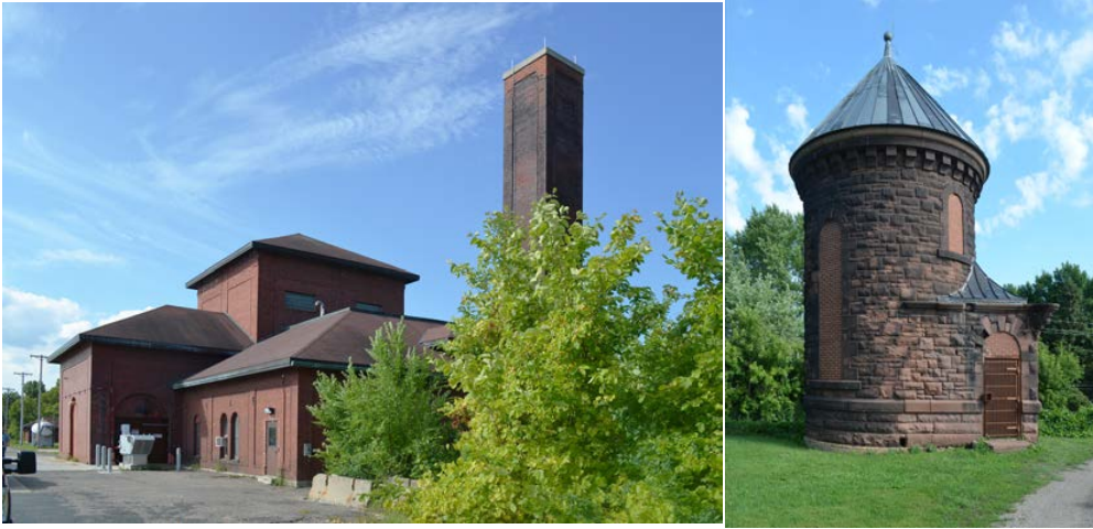
Minneapolis filtration plant and one of the three “Gatehouses” at the Waterworks.
