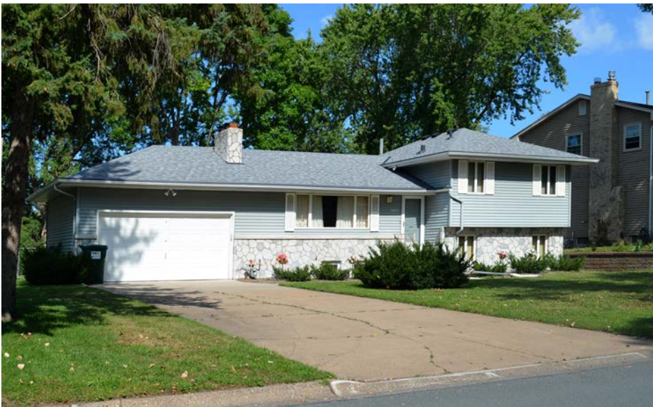
Another example of the Split Level Ranch is seen at 1421 Lincoln Terrace.
