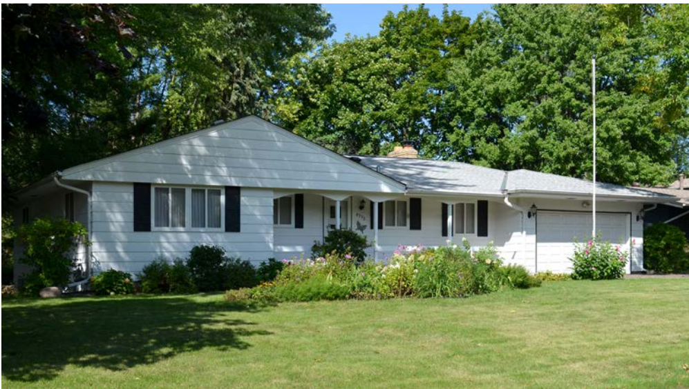
This Ranch House is located at 4990 Johnson Street.
