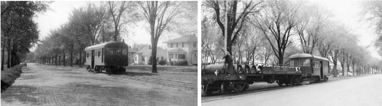
The first photograph shows the Minneapolis Filtration Plant Railway streetcar on its dedicated rail line that ran up the west side of Reservoir Boulevard from the Soo Line interchange just south of 37th and Central Avenues NE. The second photograph, taken in 1951 by Herman Rinke shows the streetcar and flatcar heading southwest on Reservoir Boulevard after a deliver of liquid chlorine to the Minneapolis Waterworks filtration plant. These historic photographs are from the Minnesota Digital Library contributed by the Minnesota Streetcar Museum.
